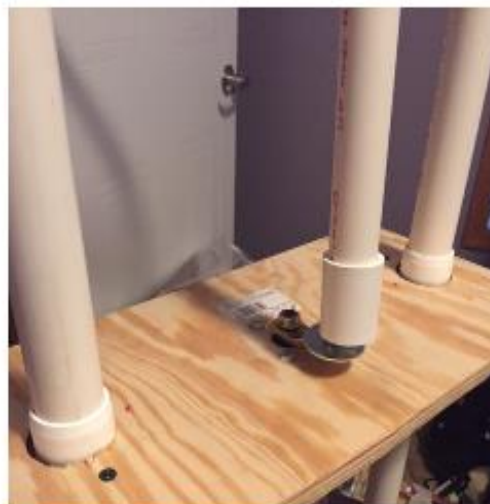
Added a 1" wood screw into the T's to mount wood base.
